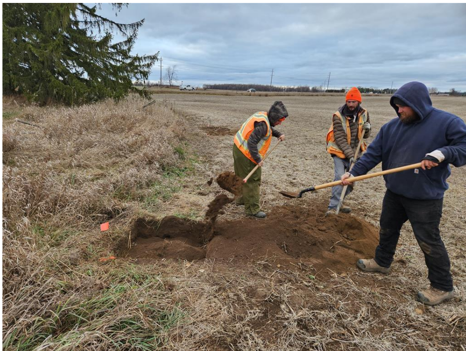
Image 4: Backfilling in progress; facing north, November 14, 2022.
